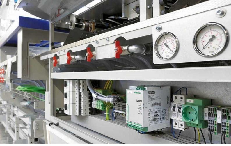
Figure 1 I Kolbus GmbH & Co. KG from Rahden (Germany), a market leader in the area of bookbinding machines, deploys multiple distributed power supplies located at the main load points.
