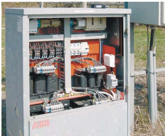
Kabeldon enclosure used for control equipment for adjustment of roundabout illumination at the entrance to Kalmar (E22), Sweden.
