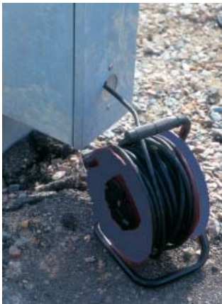
The openings on the sides of the cabinet is used for temporary power outlets, etc.
