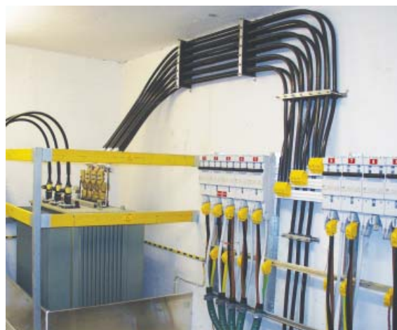
Kabeldon low voltage products mounted directly on a wall in a substation in Trondheim, Norway.
