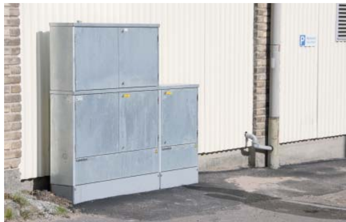
Cable distribution board in Malmö, Sweden.
