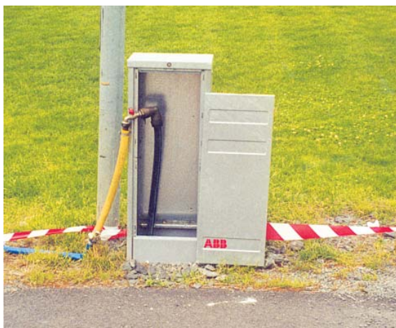
In Jönköping, Sweden, a CDC enclosure has been used for the water supply for the trade fair site.
