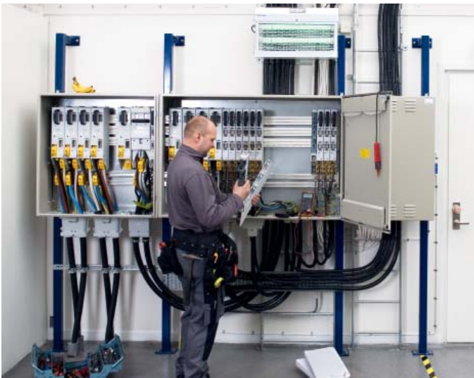
Cable distribution board in powder coated enclosure mounted on the wall at the bakery shop in Gothenburg, Sweden.
