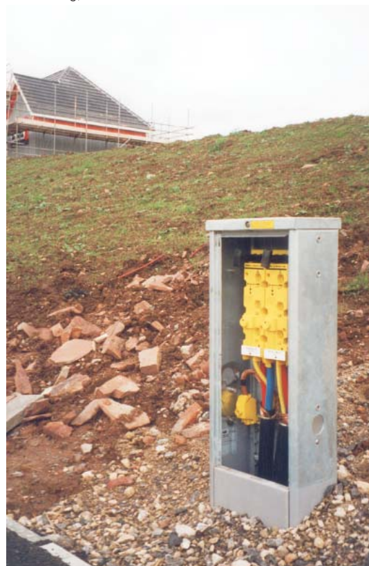
Junction box installed in Bristol, England. This replaces the conventional underground junction box.
