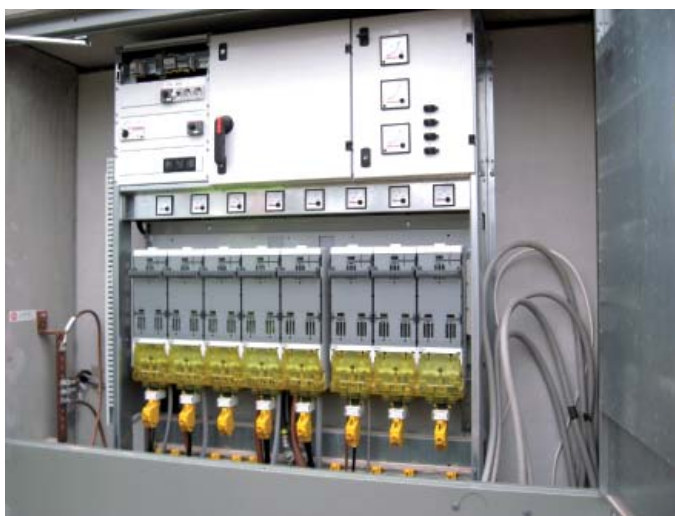
Kabeldon switching devices in a switchgear.
