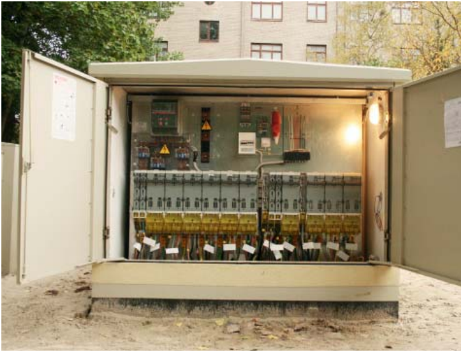
Kabeldon switching devices in substation distribution, Latvia.
