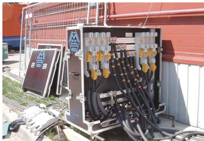
Temporary service distribution boards for the "Eurovision Song Contest 2003" in Riga, Latvia.
