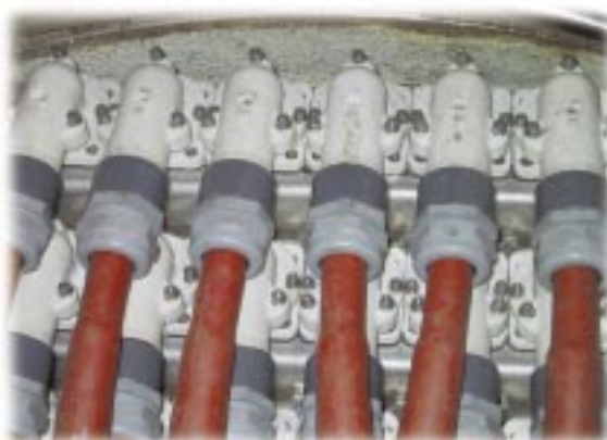
Cavotec single pole 6kV connectors
