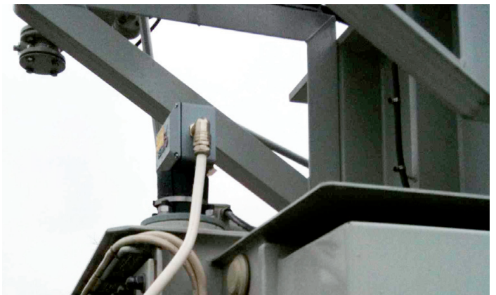
Temperature switch monitoring internal oil temperatures
