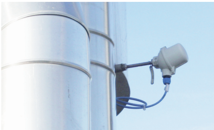
Temperature measurement of a process gas with temperature sensor TSP131
